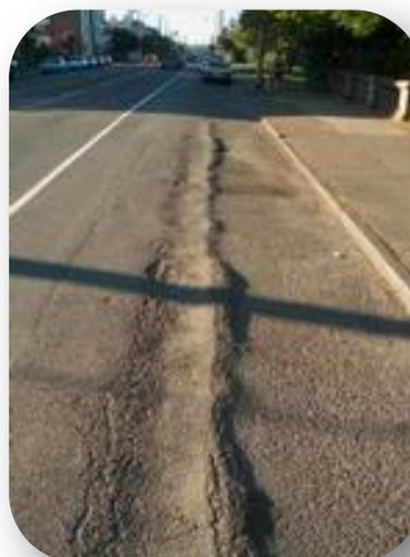
Figure 1-b: rutting in the effect of applying additional load.
