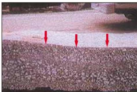
Figure 3: Deformation of pavement before substitution with SMA admixture along with iron slag.
